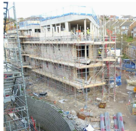
East block under construction
