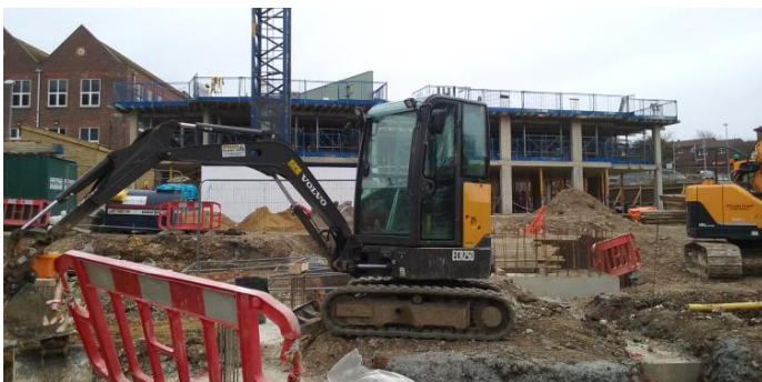
Work underway at Hobby Place
