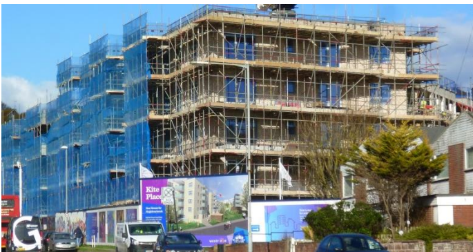
West block under construction
